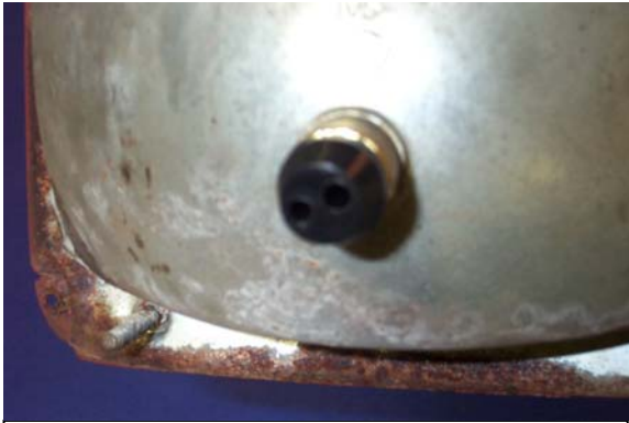
The supplied wire guide successfully installed in the bulb socket.
